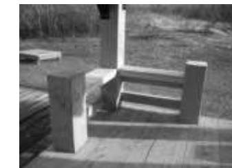
Detail of new Whistlestop shelter at Spencer
